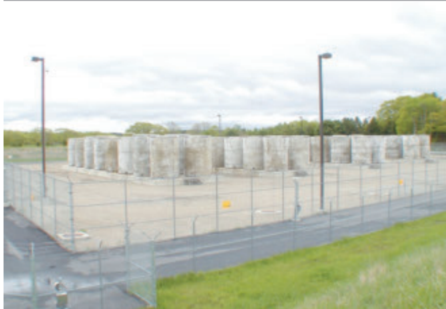
FIGURE 14. DRY CASK STORAGE FACILITY AT THE DECOMMISSIONED MAINE YANKEE REACTOR SITE
