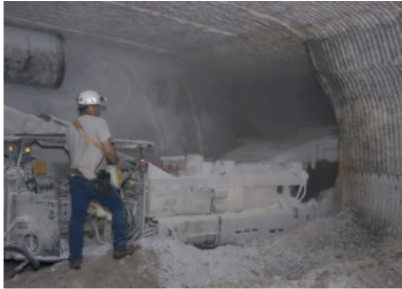
An underground chamber at the WIPP facility.
